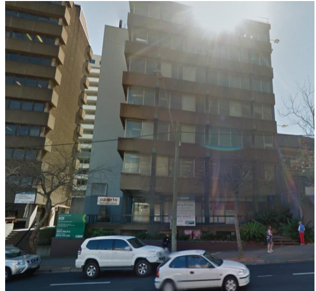
Picture 2 – 617-619 Pacific Highway
