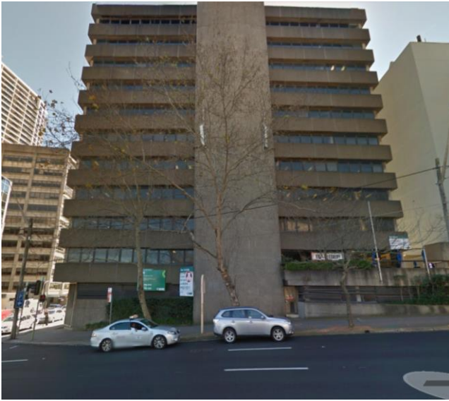
Picture 1 – 621 Pacific Highway
